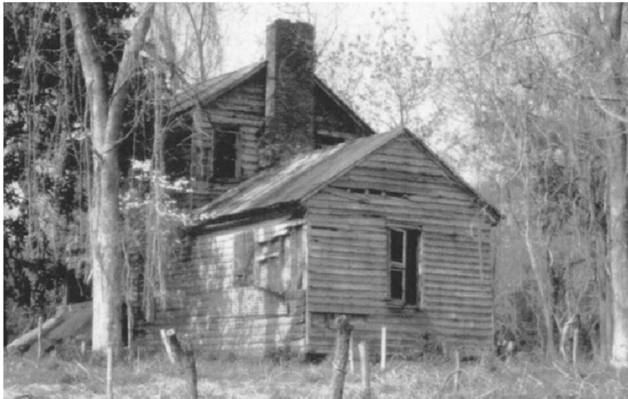
Photos are courtesy of Homer Buck who demolished the old house
