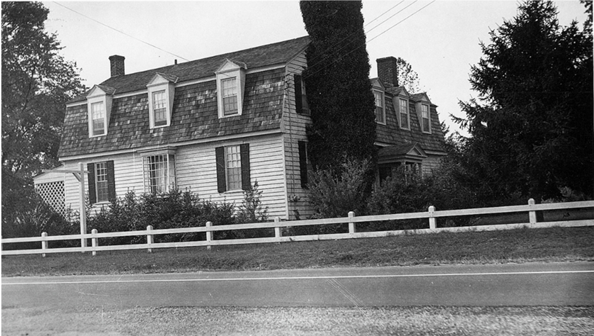
Photo dated 1953 – before the building was moved back and rotated
