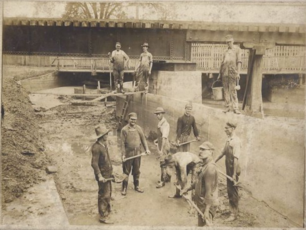
DRAINAGE DITCH OUTSIDE BROOKSIDE MILLS
