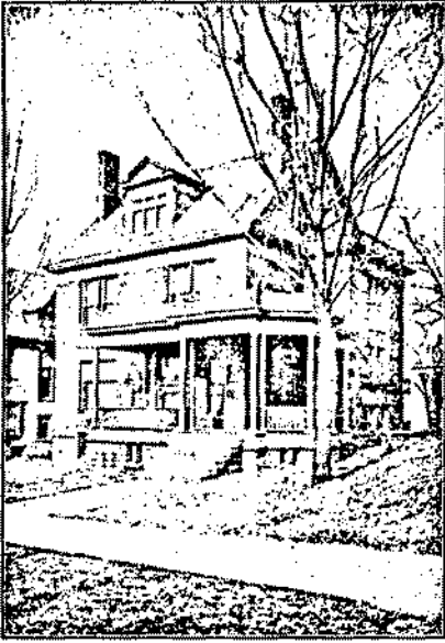
RESIDENCE OF EDWIN M. LONG, LINCOLN AVE.
