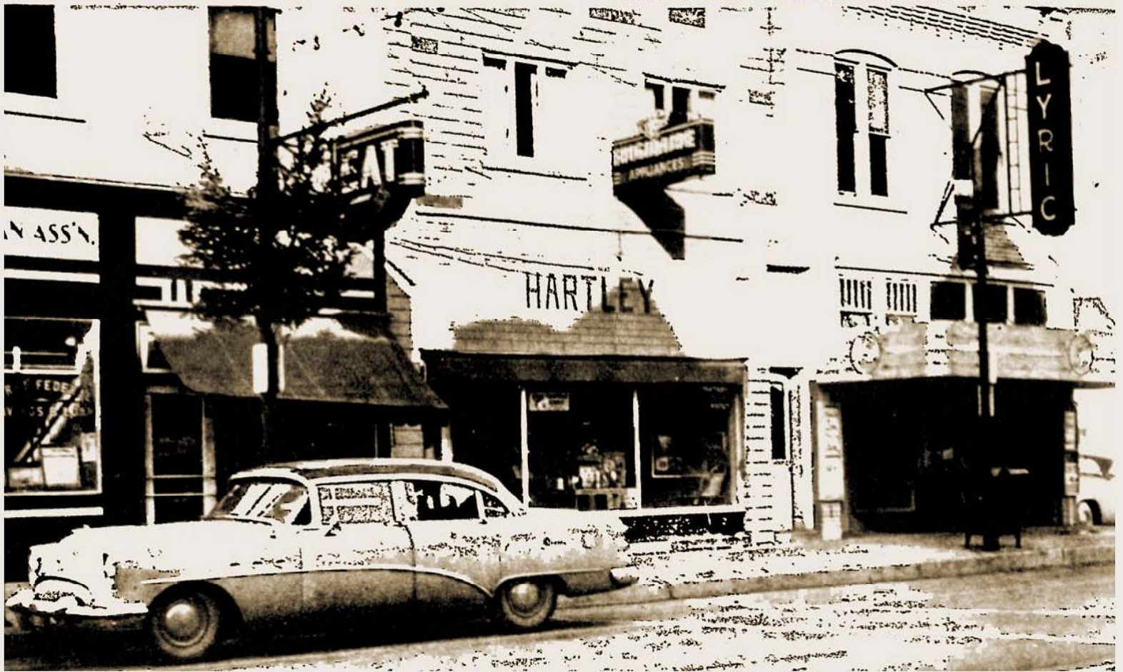
SEVERAL STORES, a theater, a restaurant and a savings and loan association are across the street from the bank
