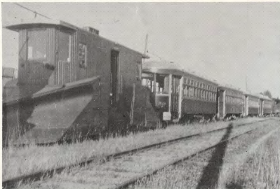
WAITING for the junkman's torch is this lineup of cars on the siding at the old Fairgrounds after abandonment of the Waterville, Fairfield & Oakland Railway in 1937. — [Photo from Lloyd McAuley.
