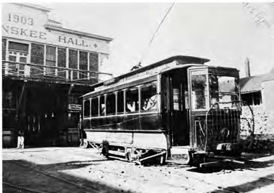
EX-BOSTON ELEVATED car No. 16 at the Oakland car-house about 1911. The car was built by J. M. Jones' Sons of Watervliet, N. Y., in 1892 by lengthening a 16-ft. horse-car.—[Courtesy Wm. Gagnon.]
