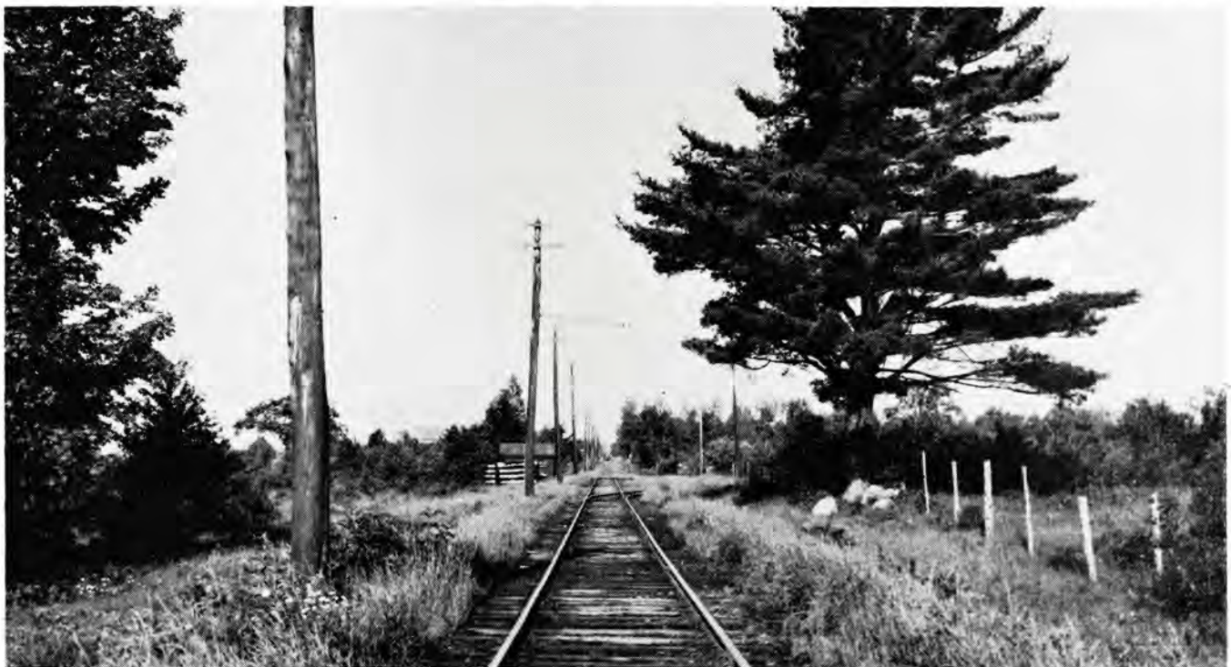
TYPICAL SCENE on the cross-country Oakland line—a 1935 view at Rangeway turnout, Birney car in distance.
