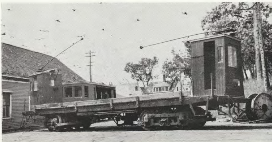
MOTOR FLAT CAR No. 1, built on the underframe of Stephenson 14-bench open car No. 1, at the Fairfield barn.
