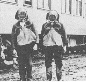
Early mine rescue gear to allow into hazardous atmospheres. Behind is a special mice rescue railroad car operated by the US Bureau of Mines Courtesy Black Diamond Historical Society
