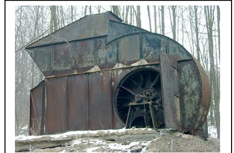
This fan is still extant at the site of Johnstown Coal and Coke's coal preparation complex at Allendale, PA.
