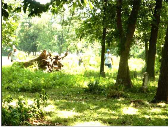
LEFT – This photo was taken at the beginning of the clean-up. A large dead tree has fallen over but has not damaged any of the stones.
