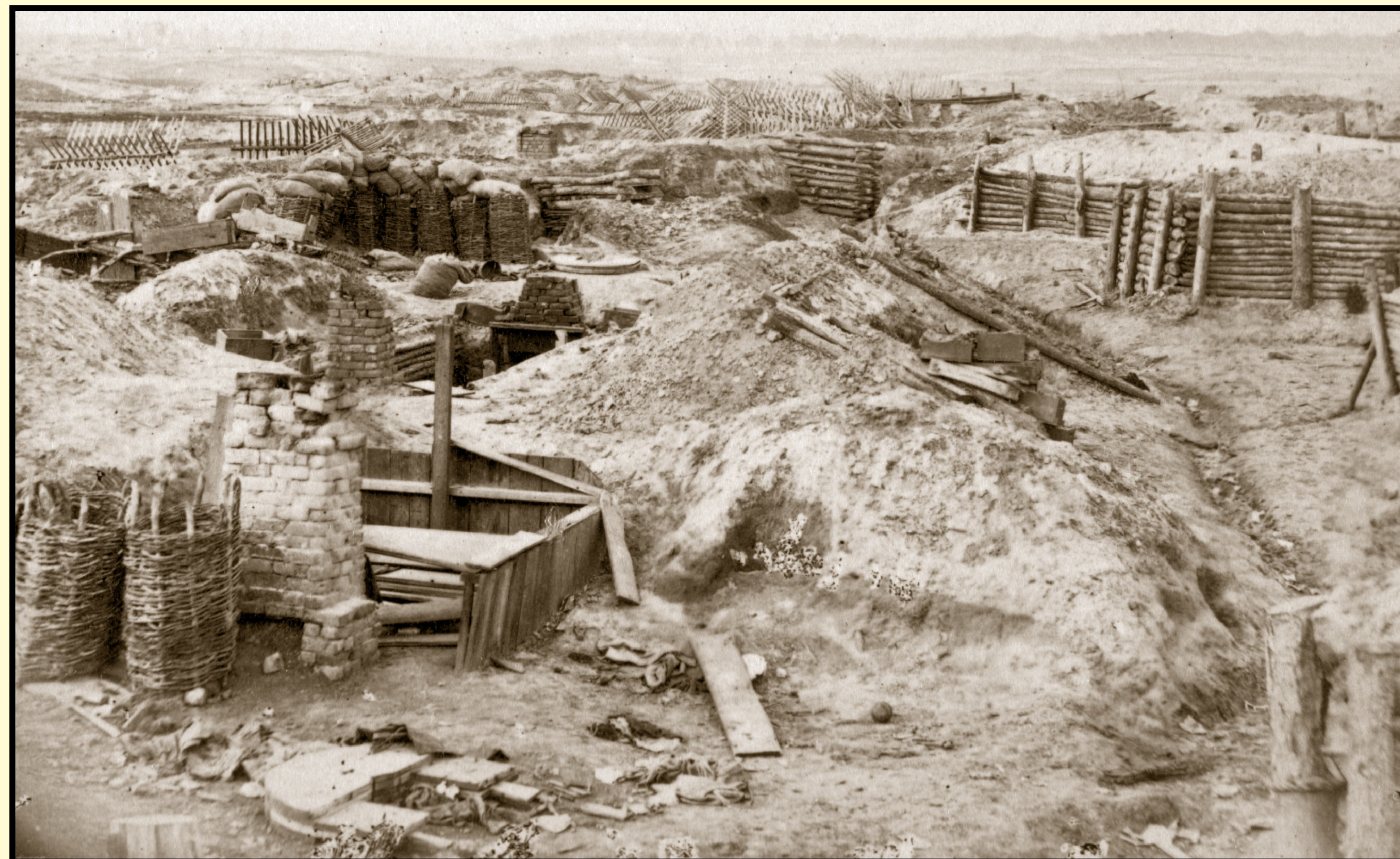
Gabions and log earthwork construction – Courtesy Library of Congress
