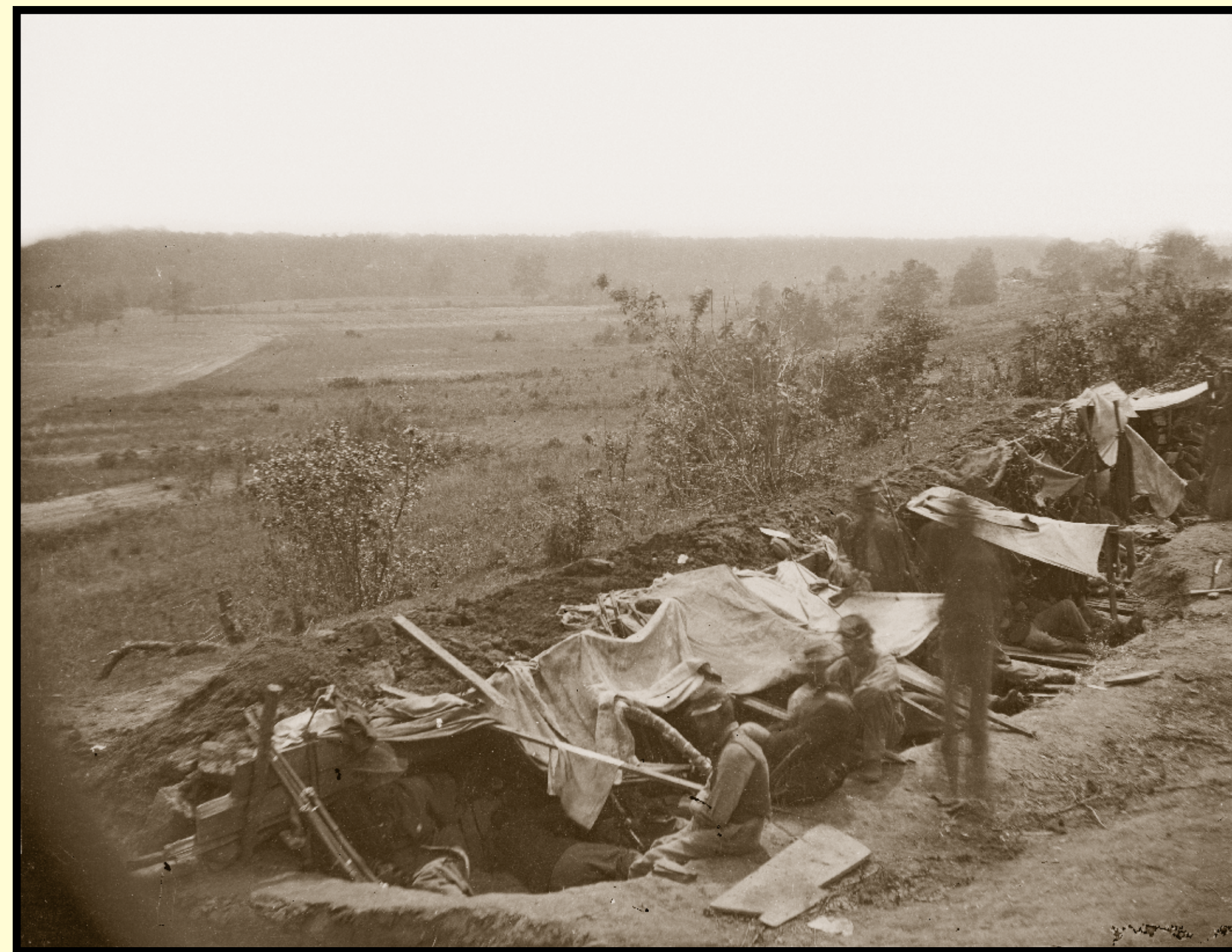
Breastworks such as these protected the soldiers, who stood upright against the wall and fired over the parapet. – Courtesy Library of Congress
