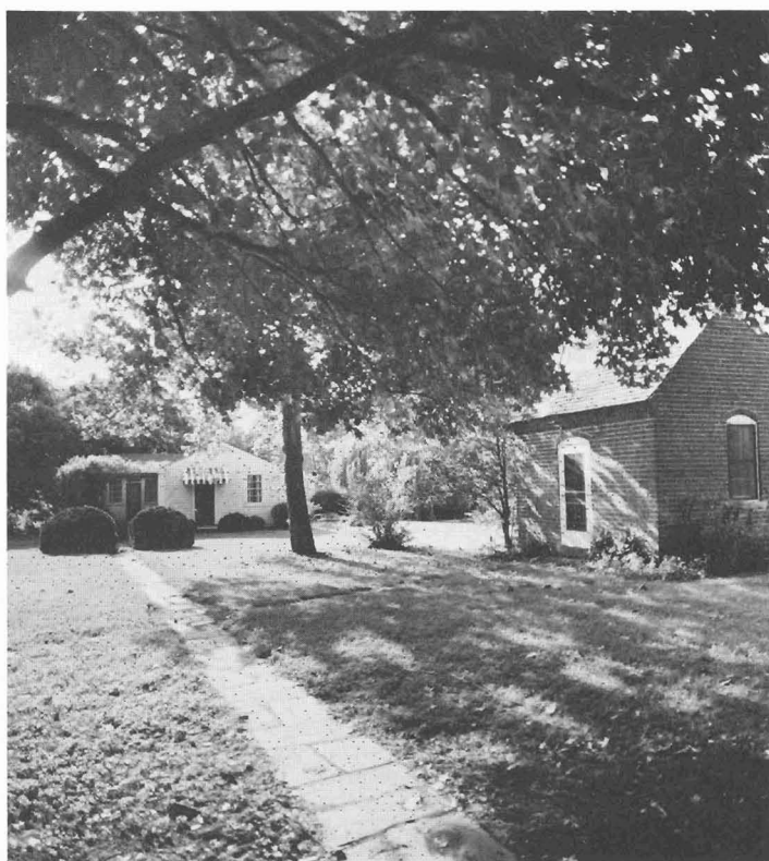
Guest house, office
