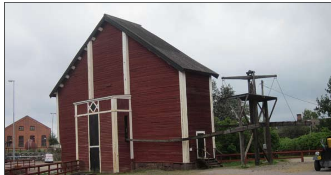
The wheelhouse for the 49 ft. Cruetz waterwheel at Falun mine
