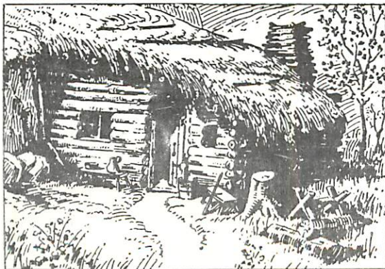
Typical Pennsylvania first settler's cabin, usually built against an earth bank to form one wall, chimney of clay and sticks.
