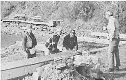
Marina repair—fall work weekend. Powers
