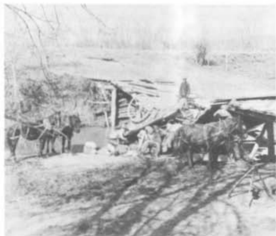
Chris Afseth on bridge, Pat McNurney in creek. Oscar Thompson resting after the accident. Notice willow tripod for coffee.
