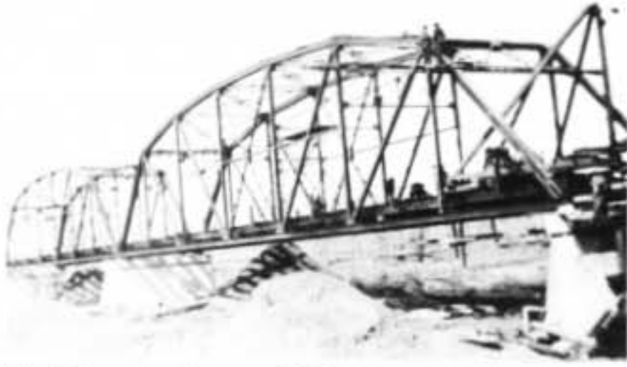
New bridge across the Musselshell River near completion in 1933
