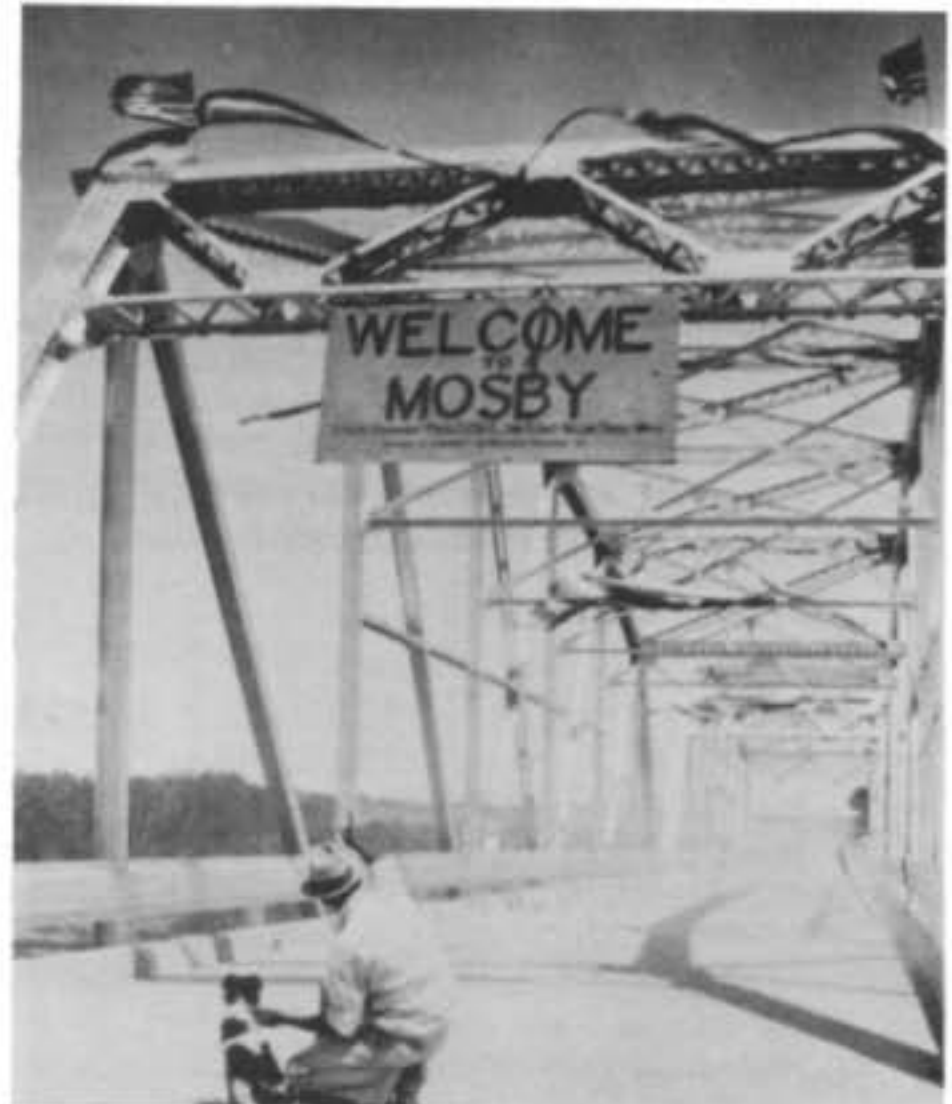
Bridge at Mosby is finished and ready for the opening dance!
