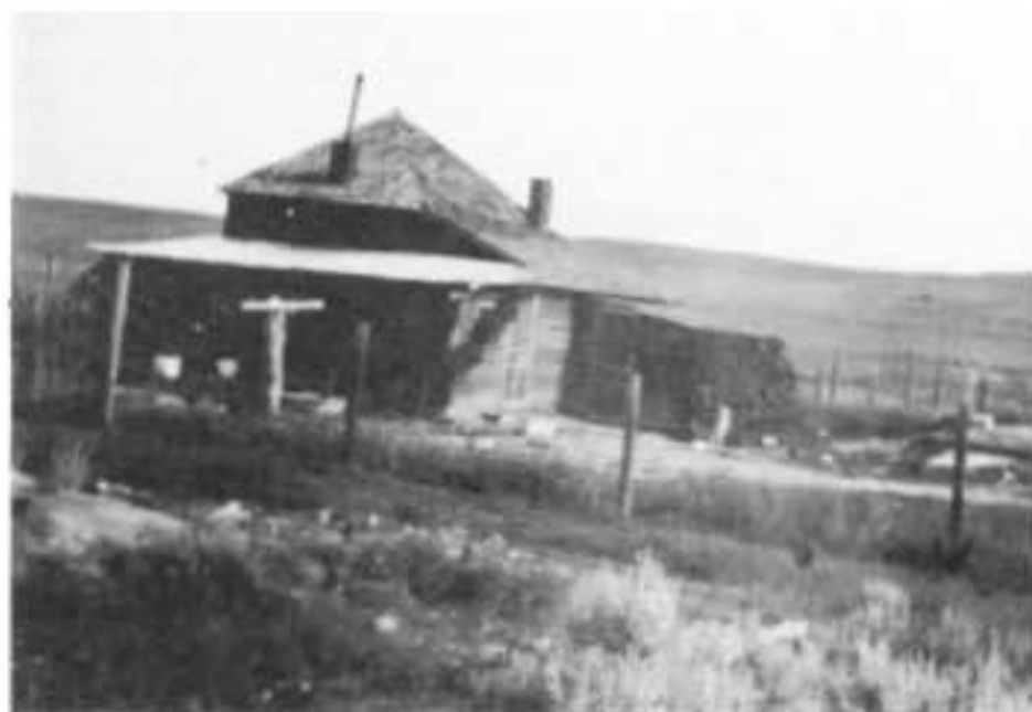
Sarvis house with additions by Munsons
