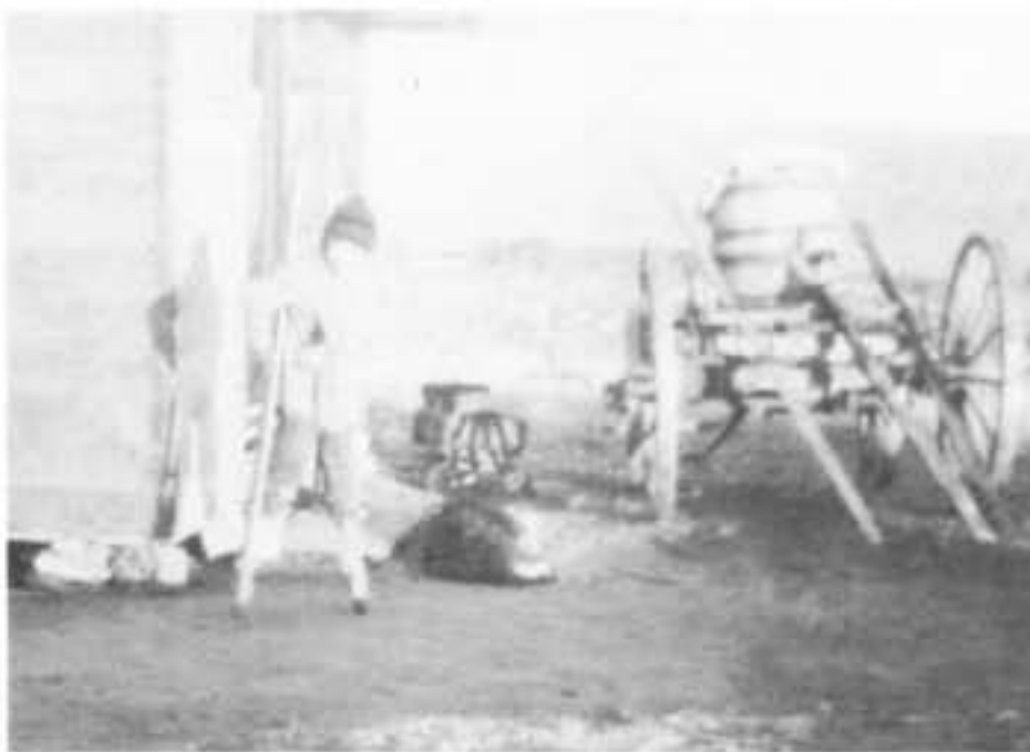
Jim Black on stilts and the Black water supply hauled from some distance
