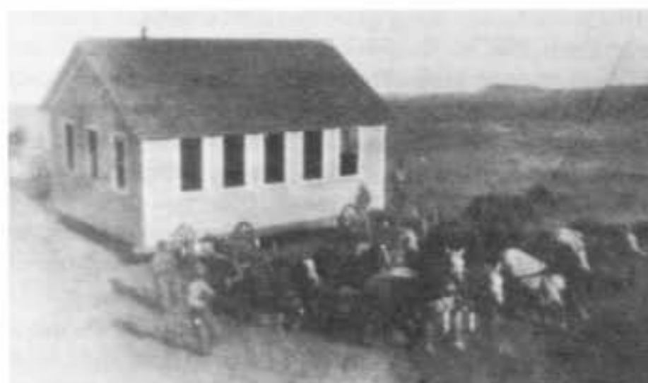
Moving the Conolly schoolhouse to the Dovetail School location
