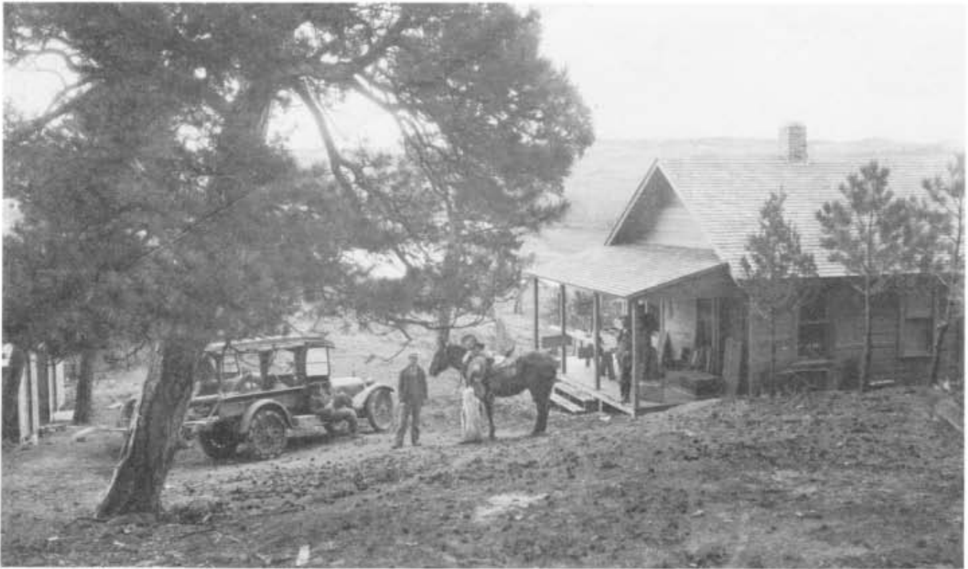
The Frantz cookhouse on the river built after the discovery was made (Photo courtesy of Montana Historical Society)
