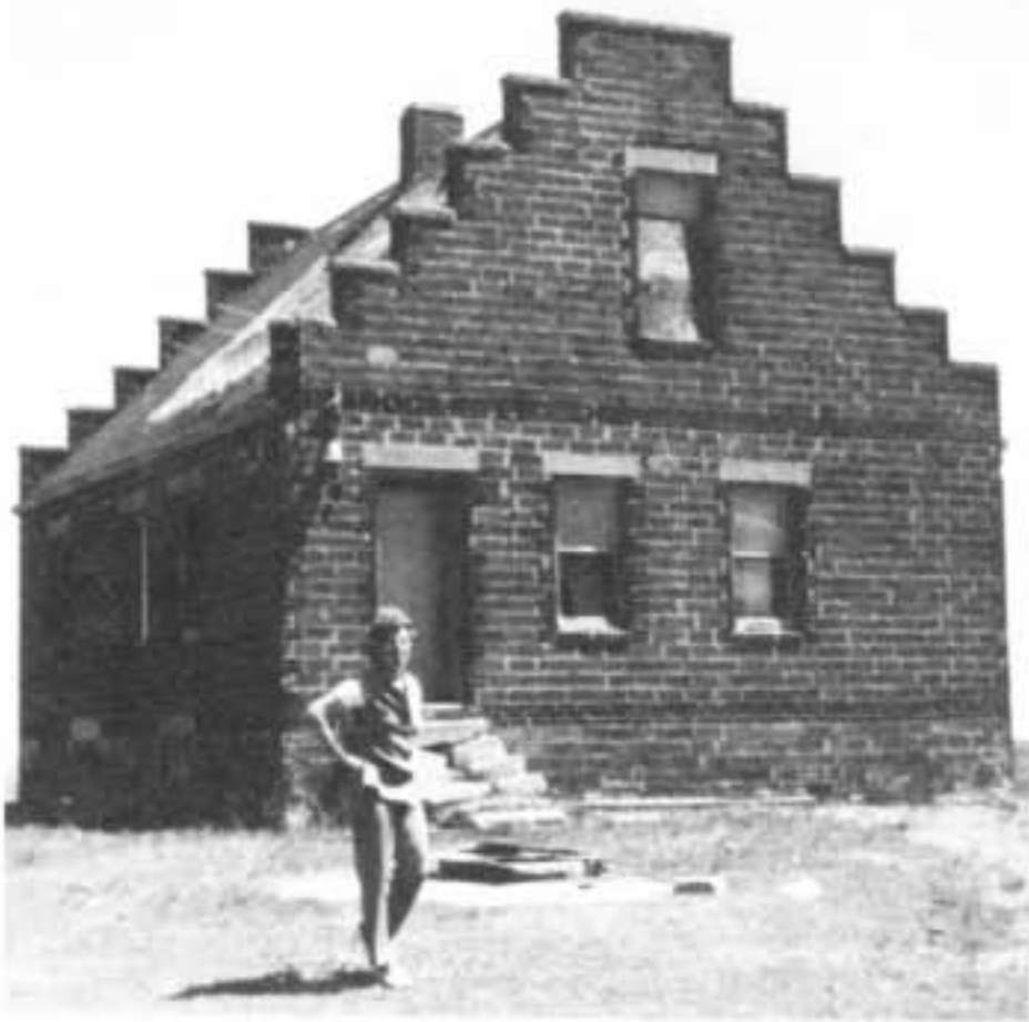
House built by Evan Holmboe. Ninnemans, Sandmans, and Stewarts were later occupants. (Picture taken in 1985)
