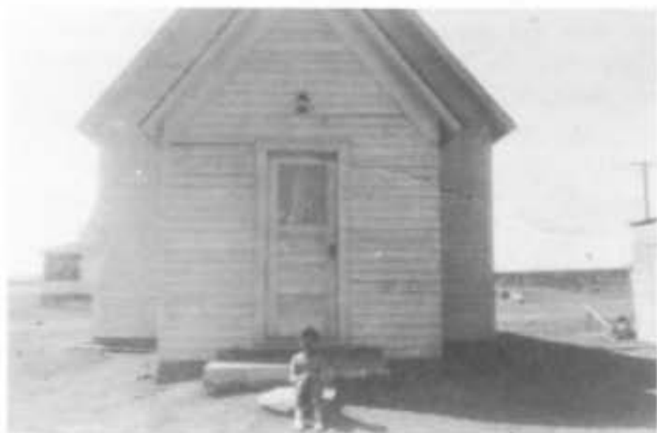
Old building moved in
