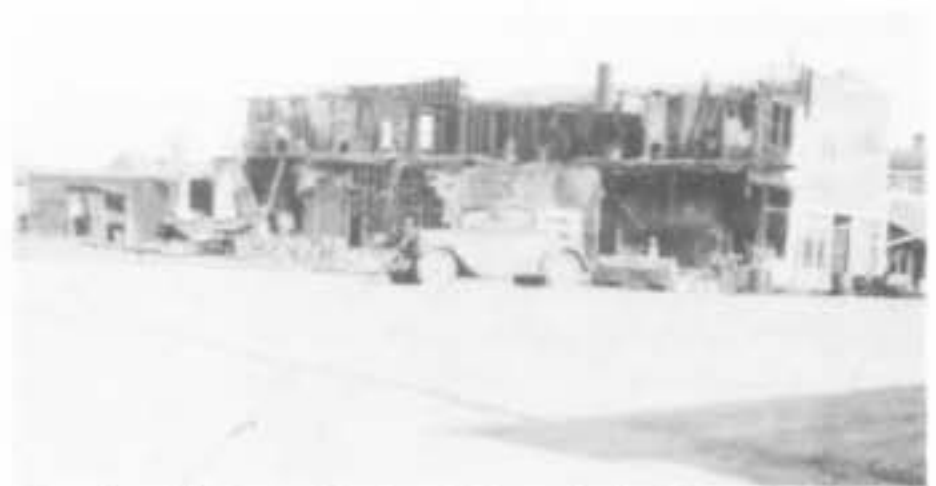
Remains of the Savoy Hotel and the two barbershops which burned in 1931. The Butte Block building and Cole's Service Station were saved
