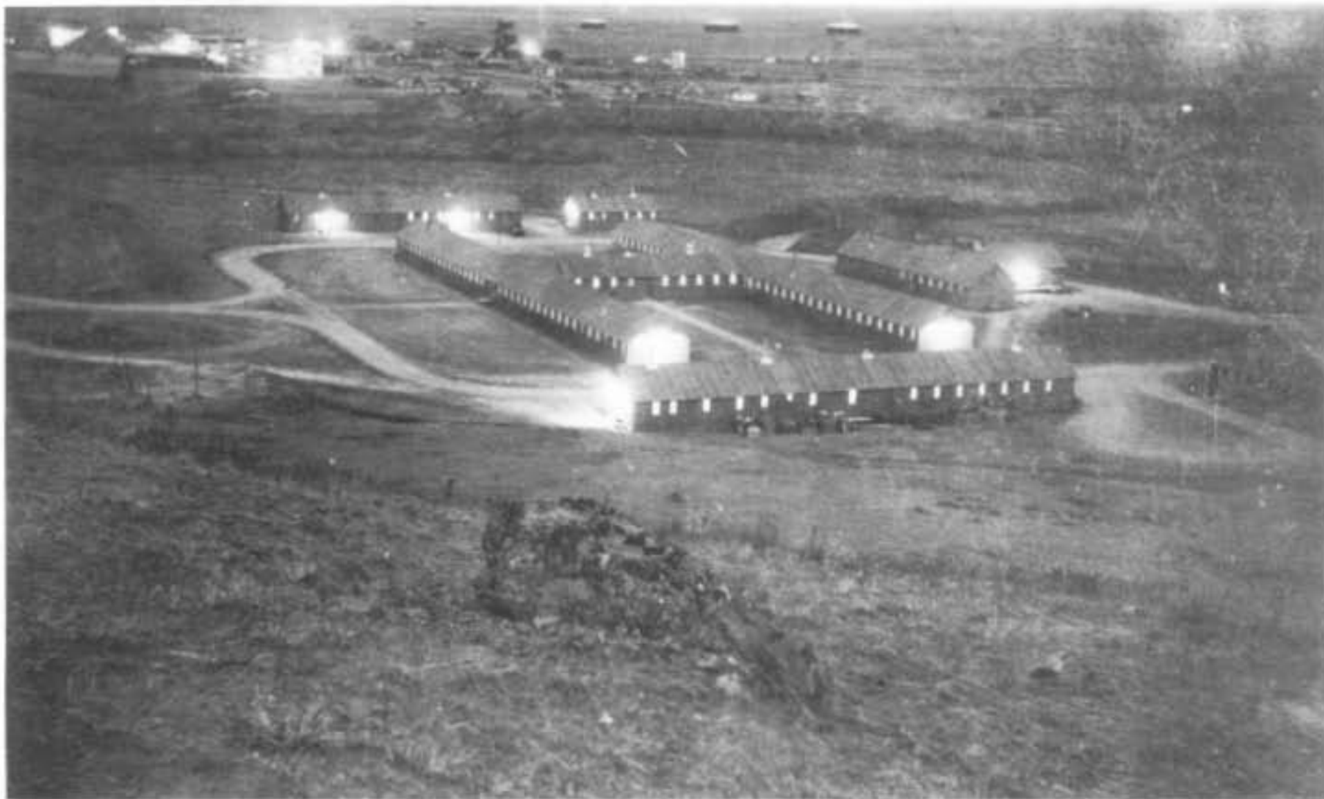
Civilian Conservation Corps camp on the outskirts of Winnett in 1936. Notice the three big black oil storage tanks on the hill!
