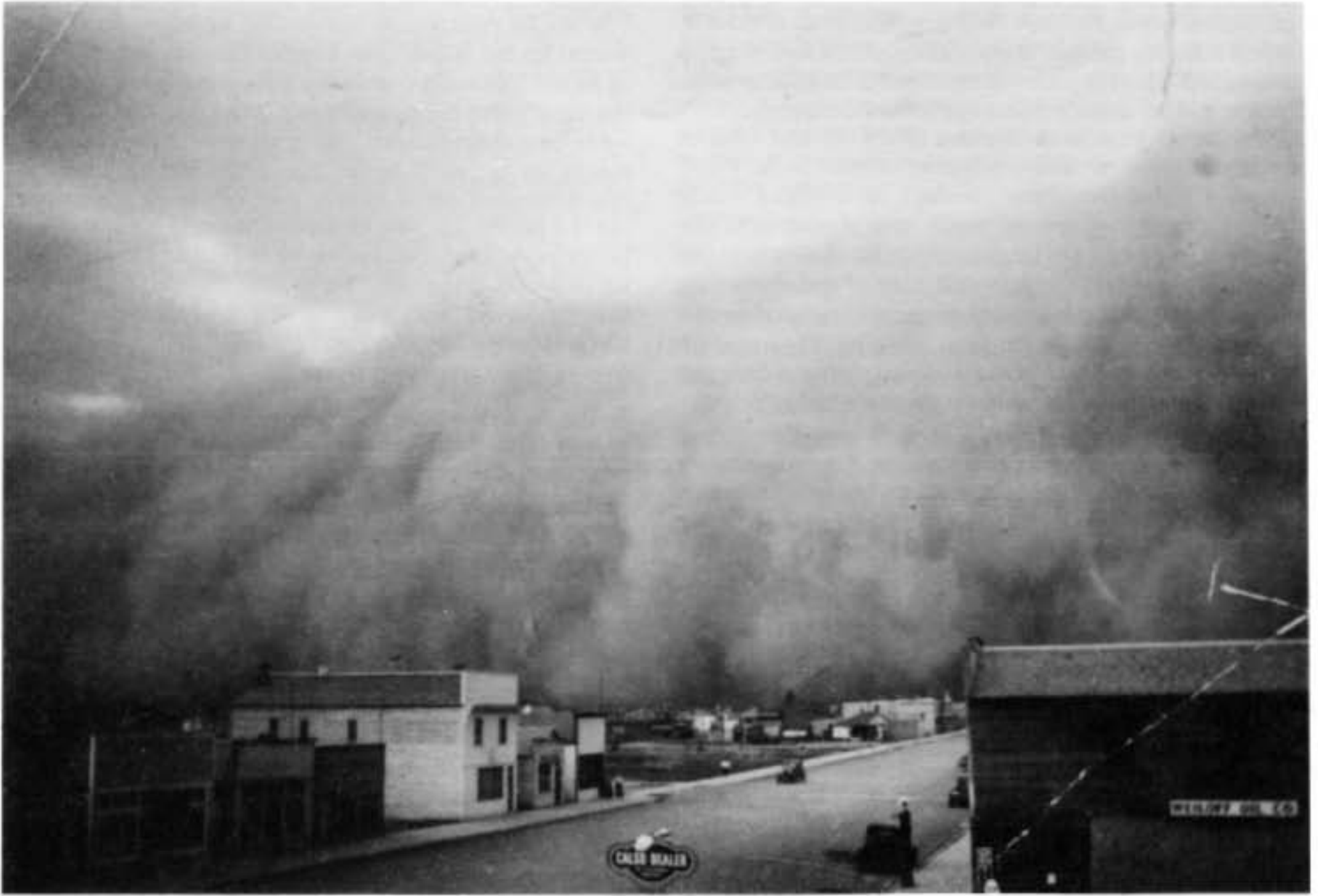
A dust cloud, reportedly created by a highway construction project, rolled into Winnett in June of 1937 and turned daylight into dusk. Shown on the south side of Winnett's Main Street are the following: (L to R) Mother Stewart's Restaurant (the original Ray Badger Restaurant which became The Mode in 1915), former Nick Langshausen office, first Winnett Times, I.O.O.F. Hall (original Moll Pool Hall), Woods Drugstore, Farmers and Merchants Bank building, burned-out Block 16, City Service Station, Winnett Post Office, Winnett Mercantile, and the rear portion of the second Aristo. On the north side of Main Street are: (L to R) Cole's Service Station, Weiloff Oil Company, and the Butte Block.
