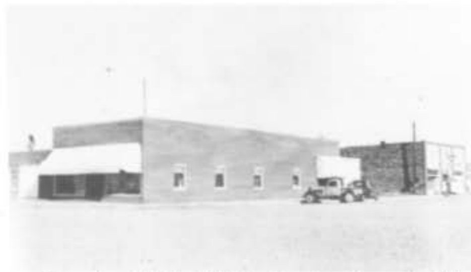
Eager store just before 1945 fire. Broadway Garage at right
