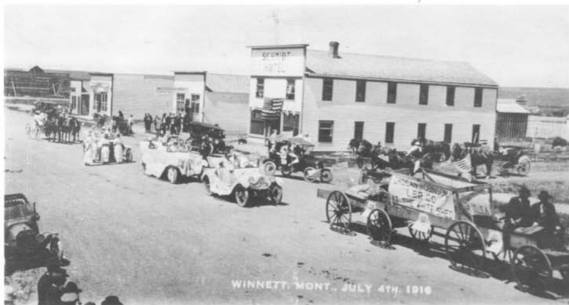
North side of Main Street in July 1916. (L to R): Eager building under construction, Bachelor Cafe, Central Billiard Parlor, Montana Bar, Schmidt Hotel
