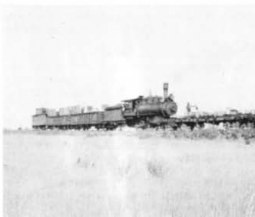
Work train laying rails between Teigen and Winnett
