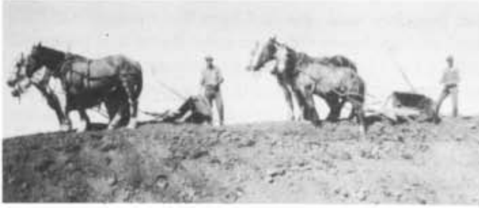
Pete Hubert and Evert Brady building roads
