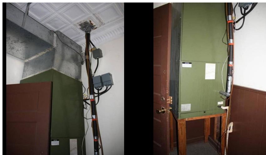
Pic 4 — Unit Located on Second Floor
