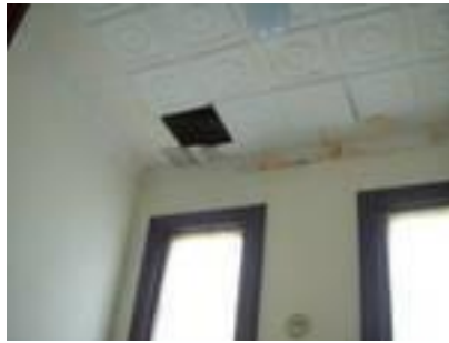
Pic 6 — Attic Access to Unit
