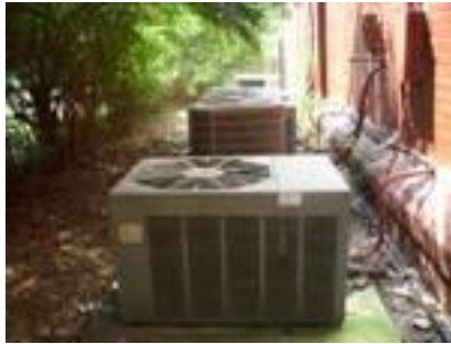
Pic 1 — East View
