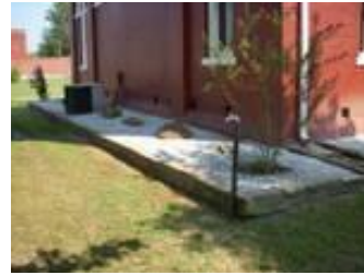
Pic 2 — West View
