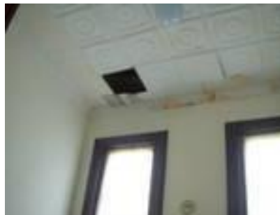
Pic 6 — Attic Access to Unit
