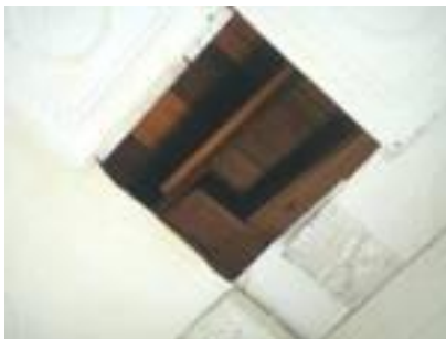
Pic 5 — Attic Access to Unit
