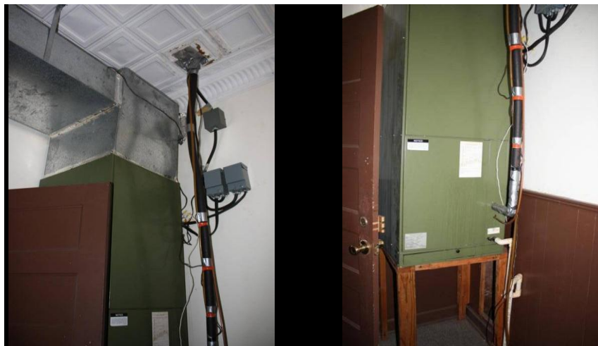
Pic 4 — Unit Located on Second Floor
