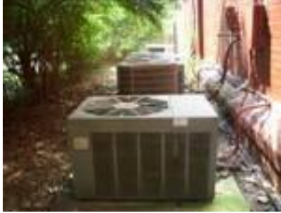
Pic 1 — East View
