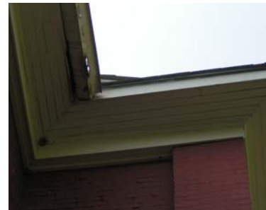
Gutter Deterioration
