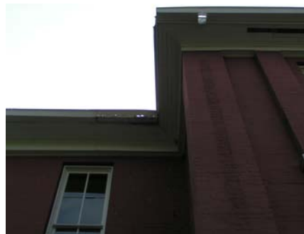
Back Gutter on Northeast Side
