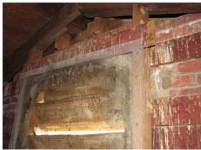
East Side of Attic
