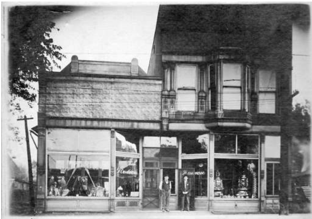
Early 1900s photo of Fickert & Kokal Hardware in Carmi, Illinois, with a full Mesker Brothers front over the original one-story building and the two-story expansion. Man on the left is Paul Fickert.
