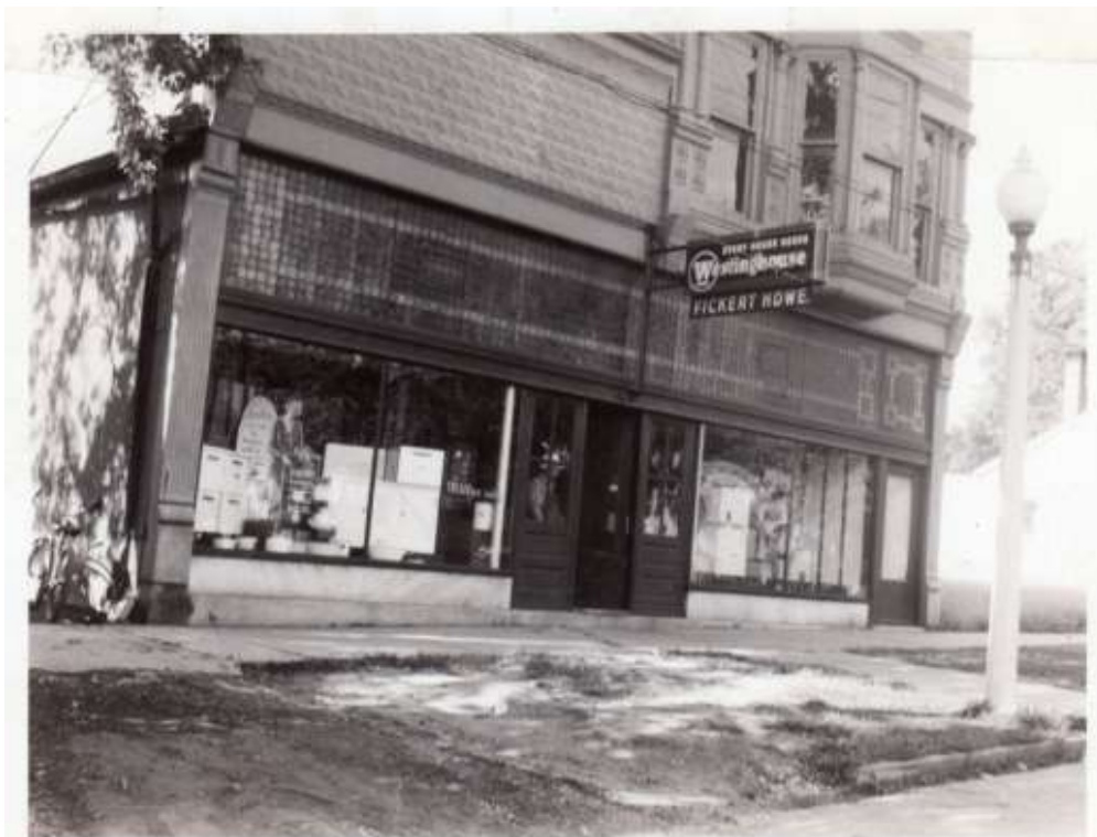
Fickert Hardware in the 1920s, with a storefront by International Steel and Iron Company and upper facade by Mesker Brothers Iron Works.
